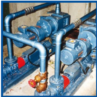
Packaged pumping system transferring raw sewage
